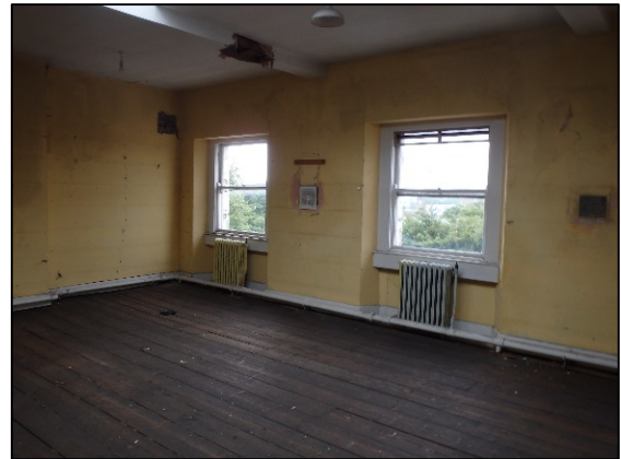
Figure 5.7.16: Example of brightly lit room in Georgian building.
