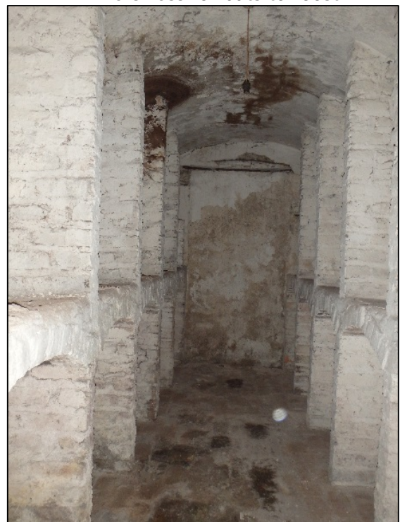
Figure 5.7.12: Cellars located within the basement of Georgian building.
